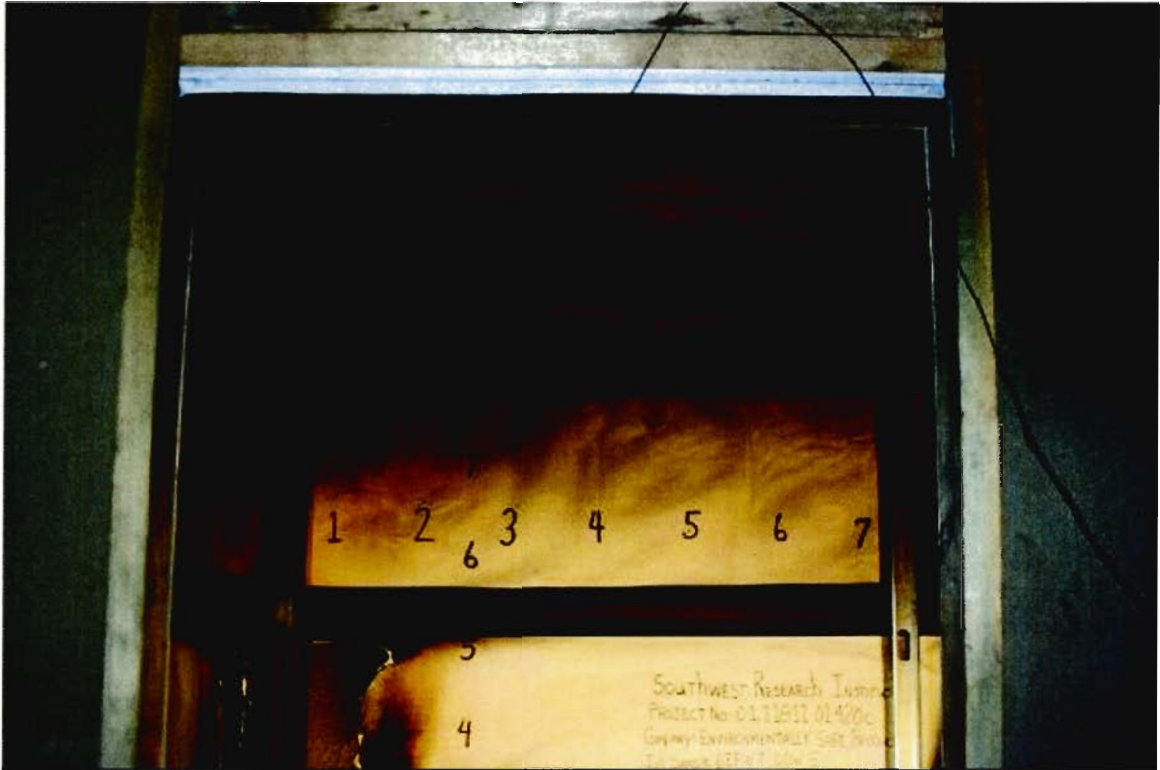
Figure B-7. Test Terminated. View of Room Interior, Back Wall and Ceiling.
